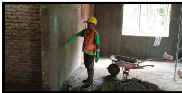
Figure 14 . Plastering work Source: Project Documentation
