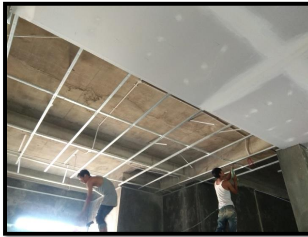
Figure 12 . Installation of Ceiling and Ceiling Frames
