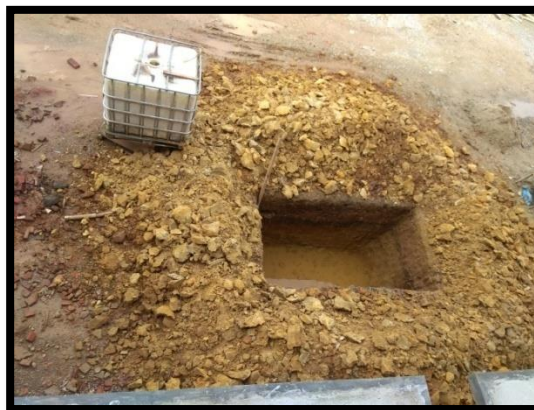
Figure 16 . Septic Tank Excavation Works
