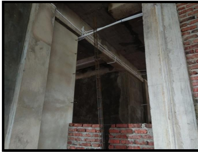
Figure 11 . Installation of Brick Cuttings
