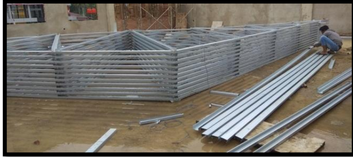
Figure 24 . Steel Easel Frame Fabrication
