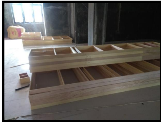
Figure 21 . Multiplex Partition Frame Fabrication
