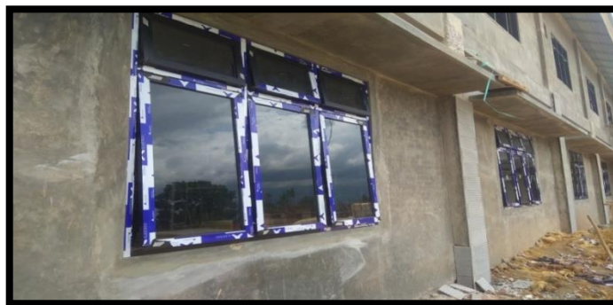
Figure 20 . Kuzen and Window Installation
