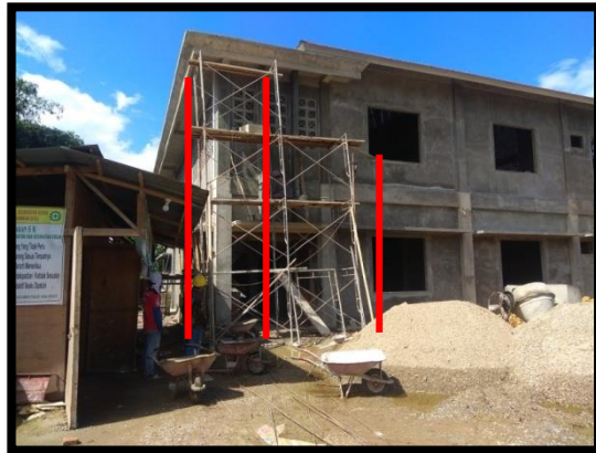
Figure 4. Inclined Scaffolding Installation Source: Personal Documentation
