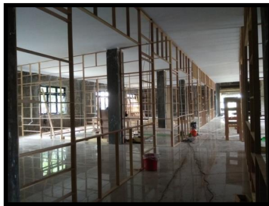
Figure 22 . Partition Wall Frame Installation
